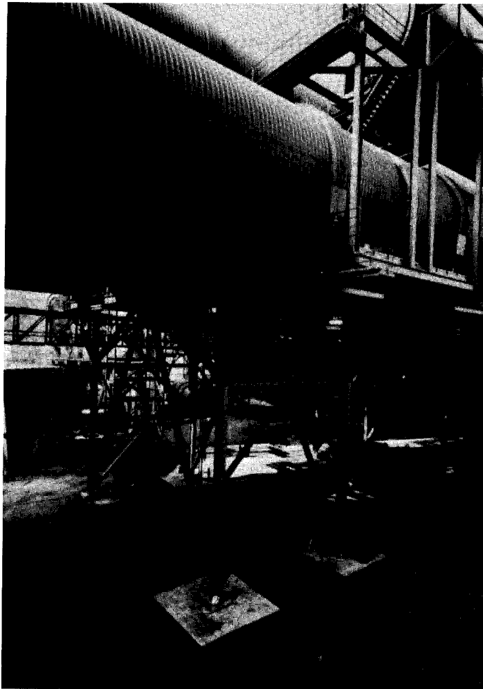
Fig. 1 Steel construction with duct loads. The support at the right in the pictures was lifted.
